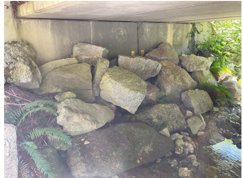
Left Bank Abutment when facing downstream
