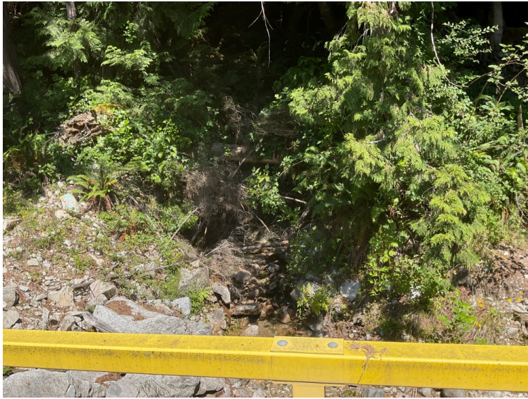
Upstream from Crossing
