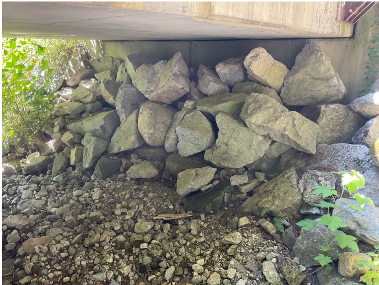
Right Bank Abutment when facing downstream
